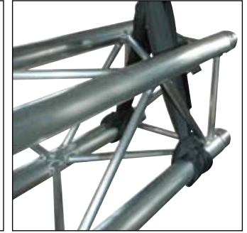
Rectangular truss 2 sling choke lower chords
