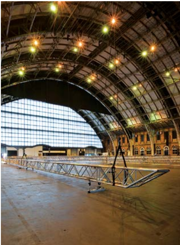
Mothergrid application at Manchester Central (GMEX) using 54 x 1.0t LoadGuard® Hoists to BS 7906: Part 1 - Category A with custom build integrated load cell monitoring and control system. Client - Litestructures for Manchester Central (GMEX).
