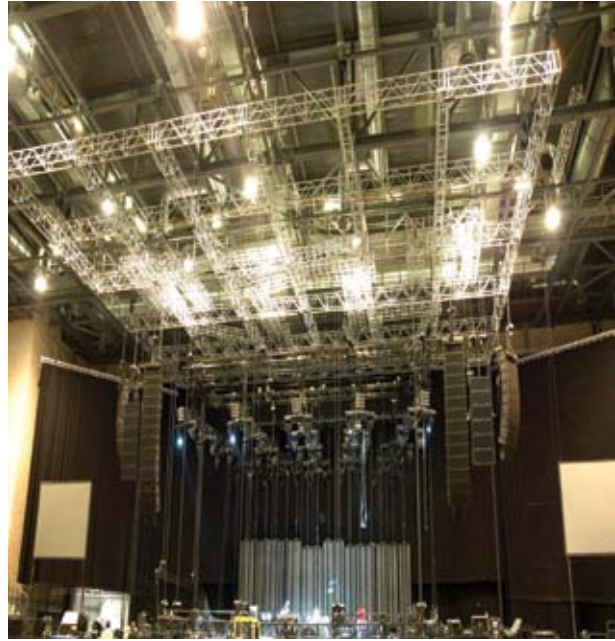
Mothergrid application at Liverpool Arena and Convention Centre using 20 x 3t SWL LoadGuard® Hoists to BS7906: Part 1- Category A, with loadcells and encoders for advanced venue safety, control and monitoring. Photo courtesy of Steve Moles. Client - Star Events Group for Liverpool Arena and Convention Centre.
