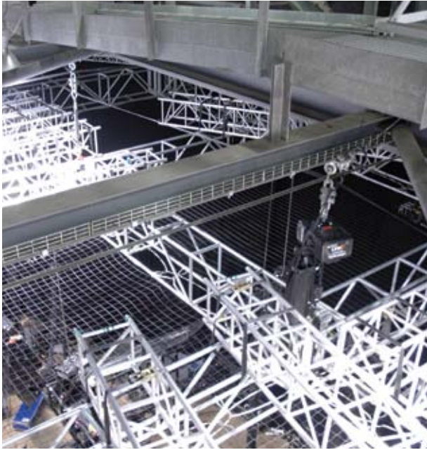
Mothergrid application at Liverpool Arena and Convention Centre using 20 x 3t SWL LoadGuard® Hoists to BS7906: Part 1- Category A, with loadcells and encoders for advanced venue safety, control and monitoring. Photo courtesy of Steve Moles. Client - Star Events Group for Liverpool Arena and Convention Centre.
