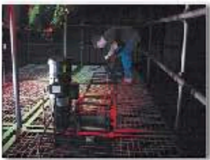
Point Hoist and Winches
